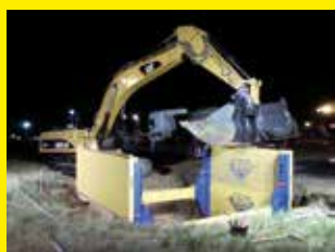
Posa in opera
